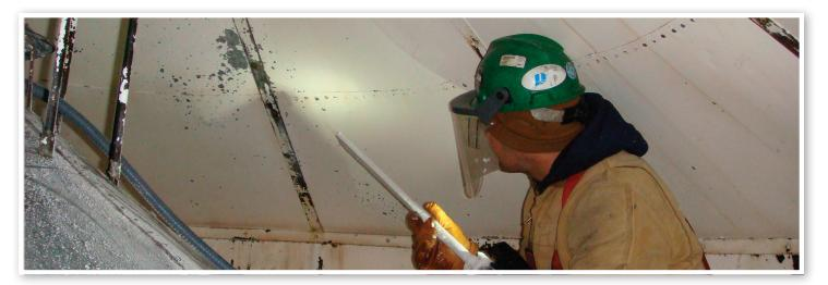
"THE GOAL WAS ONLY TO REMOVE THE LOOSE AND FLAKING PAINT, MOLD AND SURFACE CONTAINMENTS, AND PUTTY, AND WE WANTED TO DO SO WITHOUT DAMAGING THE INTERIOR OR EXTERIOR OF THE LANTERN ROOM."
