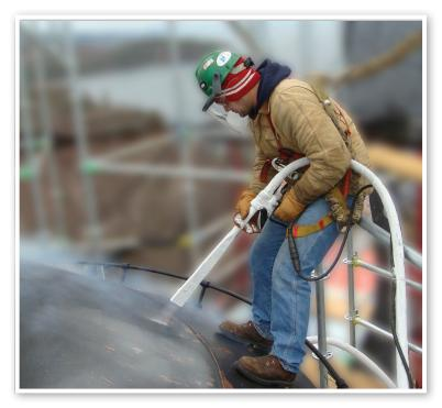
"DRY ICE BLASTING IS PROVING ITS EFFECTIVENESS IN SCORES OF CLEANING APPLICATIONS, AND THROUGH-OUT THE INITIAL PREPARATION PHASE OF THE SPLIT ROCK LIGHTHOUSE PROJECT DEMONSTRATED THAT WHEN IT COMES TO HISTORICAL RESTORATION PROJECTS, IT'S A PROCESS THAT MUST BE CONSIDERED."
